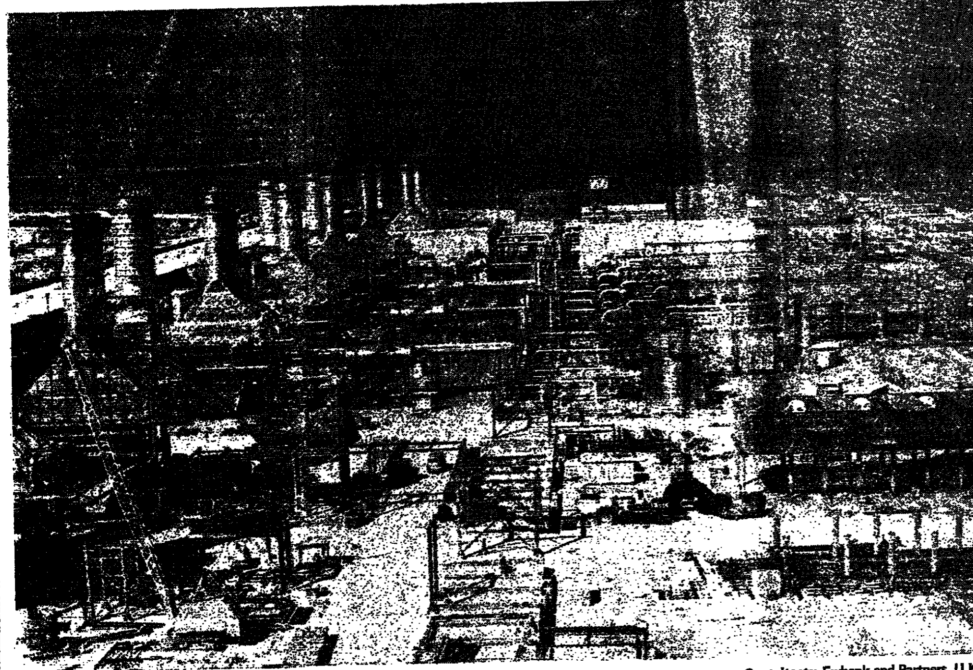
Ras Abu Fontas Power and Water Station
